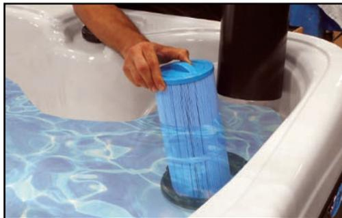
**NOTE:** Make sure the filter has soaked at least 30 minutes before you install it. Insert the filter all the way and screw it in. Do not over-torque the cartridge during installation, just hand tighten gently.
