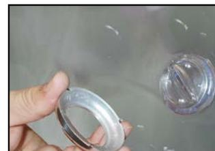
**Step 3.** Pull the plastic jet opening and its gasket off.
