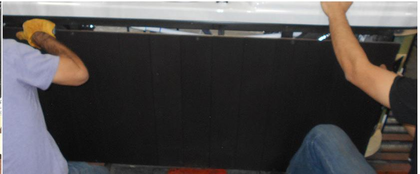
Reach in and pull the drain assembly through by a few inches. Carefully unscrew the black outer drain knob and then unscrew and remove the front door panel.
